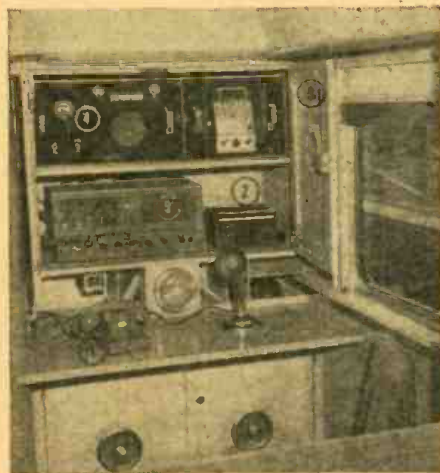
Radio Central of "The Train of Tomorrow." Radiophone handset is at (1) a control box at (2) wire recorder at (3) broadcast receiver at (4) and PA amplifier at (5). Mobile radio transmitter and receiver are in cabinet below.
